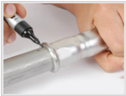
Mark the tube for reference during pressing
